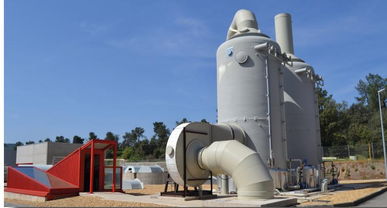
connected to an odour control system equipped with an ECOTEC biofilter consisting of two towers. This system has a treatment capacity of 68,000 m<sup>3</sup>/h.
