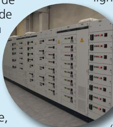
**Medium voltage system:** Internal MV ring between the WWTP transformer stations and the sectioning centre and 'CT1 PRE-TREATMENT' and 'CT2 BIOLOGICAL+SLUDGE' in existing civil engineering building, equipped with dry-type isolation transformers rated at 1,000 kVA (CT1) and 1,250 kVA (CT2), 16kV/400V-50Hz
