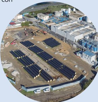
This additional thickness was required due to the construction procedures involved in the work, as the directional drilling required a reliable, safe pipe, capable of withstanding friction and stresses during the installation process. The manufacturing facilities and standards implemented by NOKSEL ESPAÑA, S.A. in the production, coating and delivery of the company's spiral-welded steel pipes always guarantee the quality and durability of each and every pipe.
